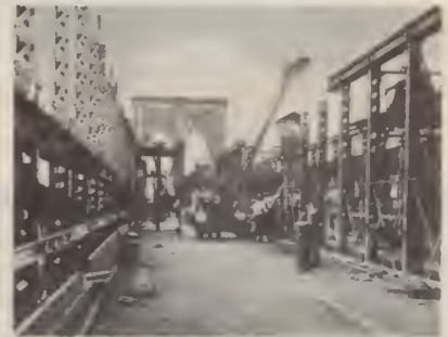
The intermediate truss was removed, right, and the top chords reused on top of the outer truss, left.
